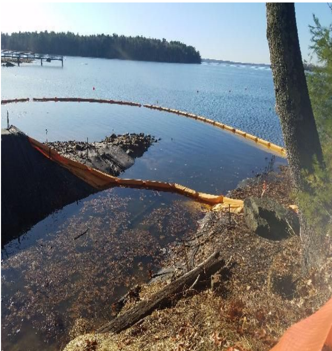
Fig 3: Silt curtains still in place at Gundalow landing/east side of the Bay. Viewing southwest. (11-21-19).
