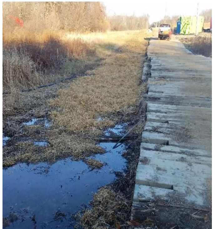
Fig 20: Straw correctly applied over wetland NW16. Viewing west. (11-25-19).
