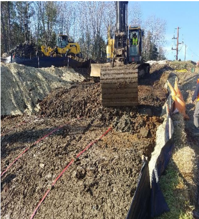
Fig 23: Backfilling trench at Getchell property/west side of the Bay. Viewing west. (11-26-19).
