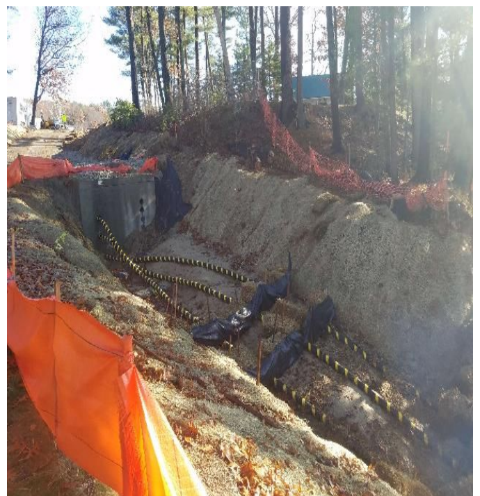
Fig 4: Vault and trench at Gundalow landing/east side of the Bay. Viewing east. (11-21-19).
