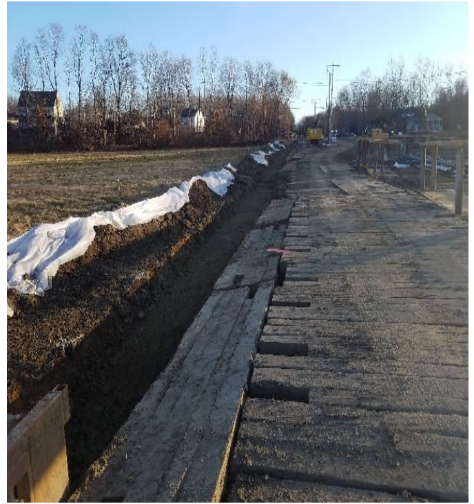
Fig 10: Trench at Frink farm. Viewing east. (11-23-19).
