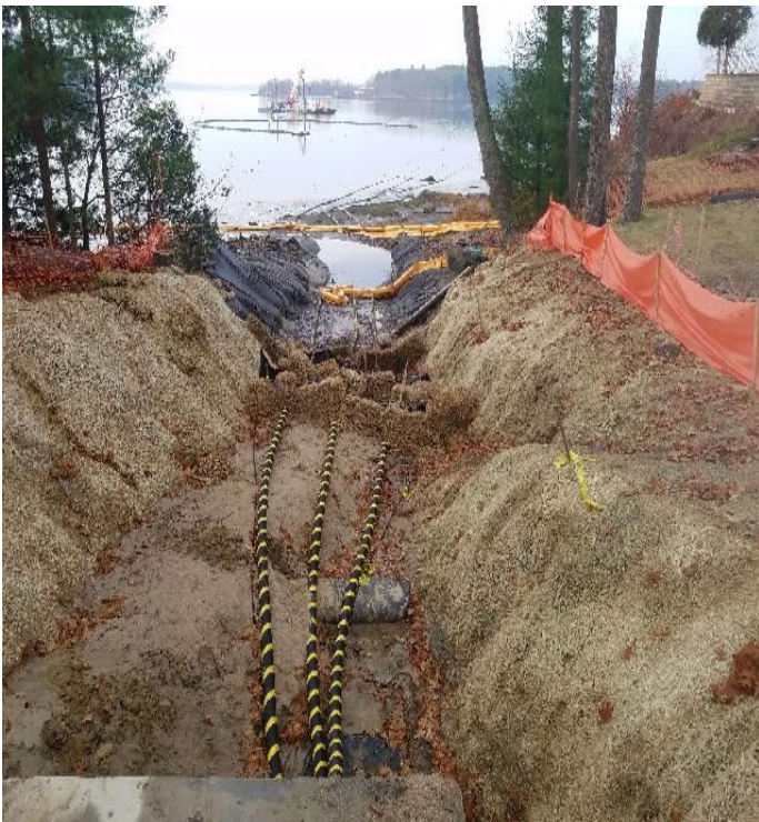
Fig 27: Trench at Gundalow landing/east side of the Bay. Viewing west. (11-27-19).
