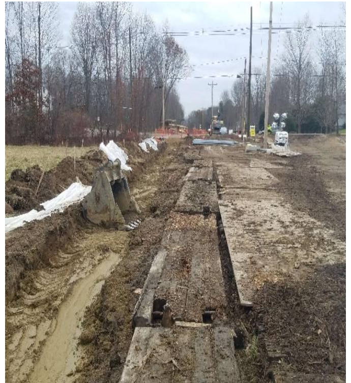
Fig 8: Backfilling soil horizons in agricultural zone at Frink farm. Viewing east. (11-22-19).
