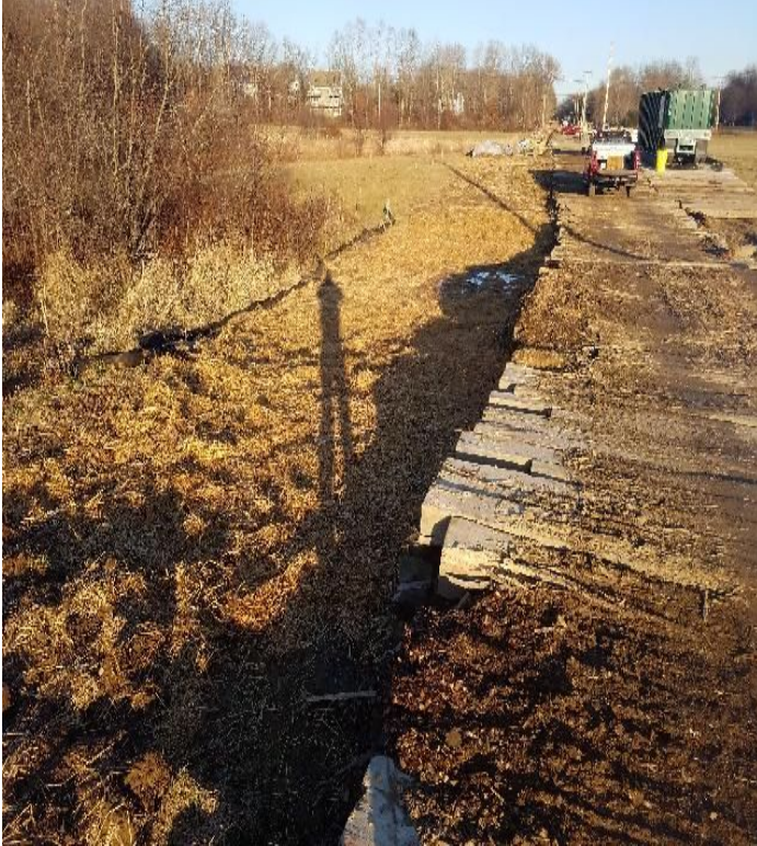
Fig 21: Straw correctly applied over wetland NW16. Viewing east. (11-25-19).
