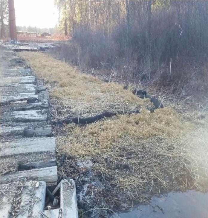
Fig 19: Straw correctly applied over wetland NW16. Viewing east. (11-25-19).
