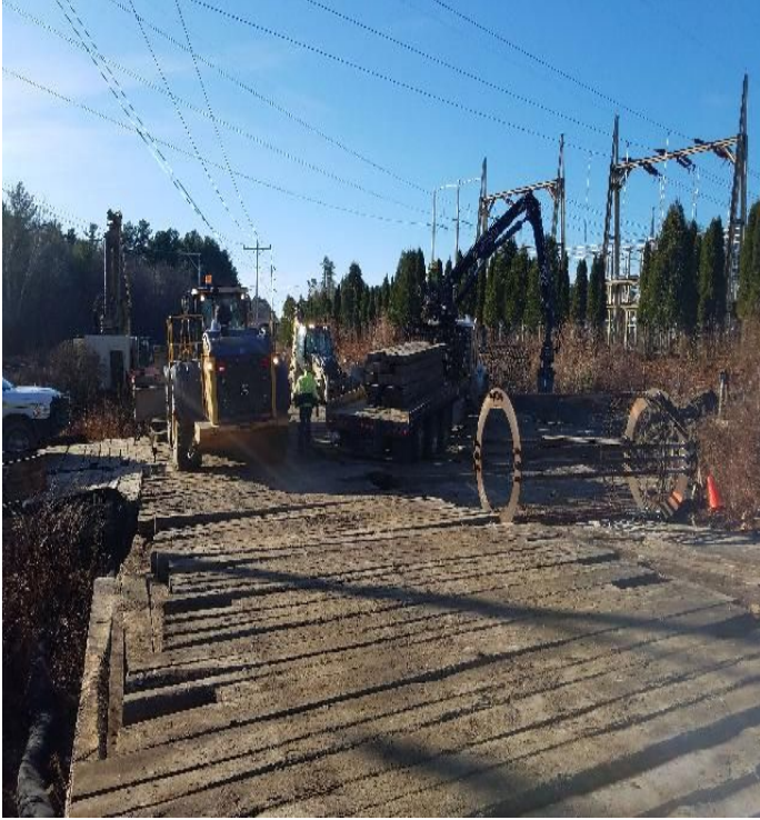
Fig 13: MJ drilling at Str. 1. Viewing south. (11-23-19). Viewing west.
