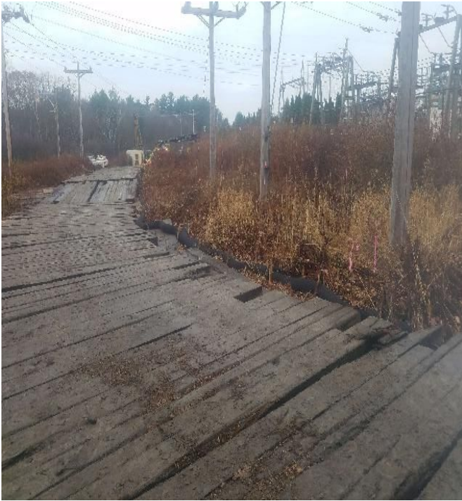
Fig 5: Filter sock installed along access road to Str. 1 and 2. Viewing south. (11-22-19).
