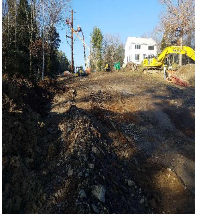
Fig 18: Backfilling trench at Getchell property/west side of the Bay. Viewing west. (11-25-19).
