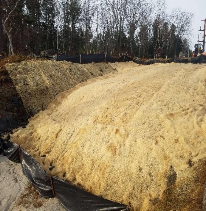
Fig 29: Temporary erosion blanket on restored slope at Getchell property/ west side of the Bay. Viewing west. (11-27-19).
