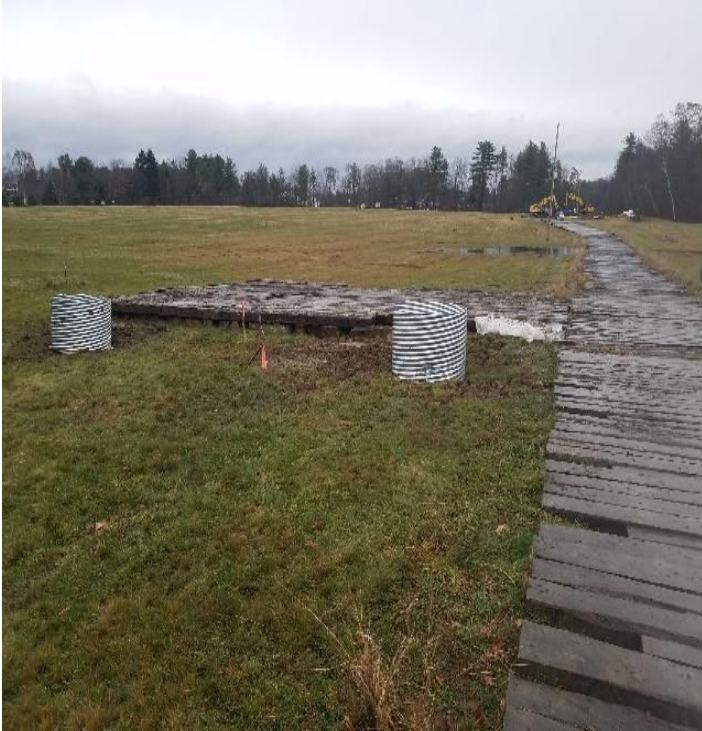
Fig 9: Direct embed foundations for Str. 110. Viewing east. (11-22-19).
